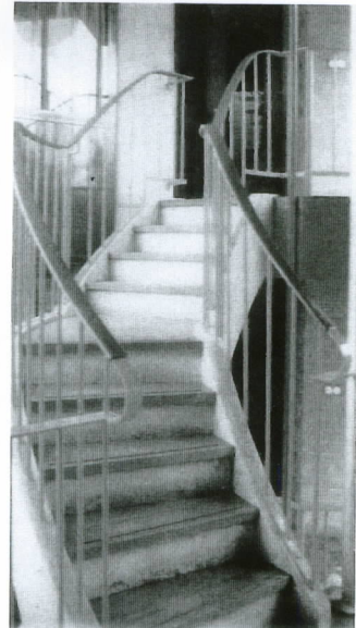
3) Mother's House, Amsterdam; stair detail.
